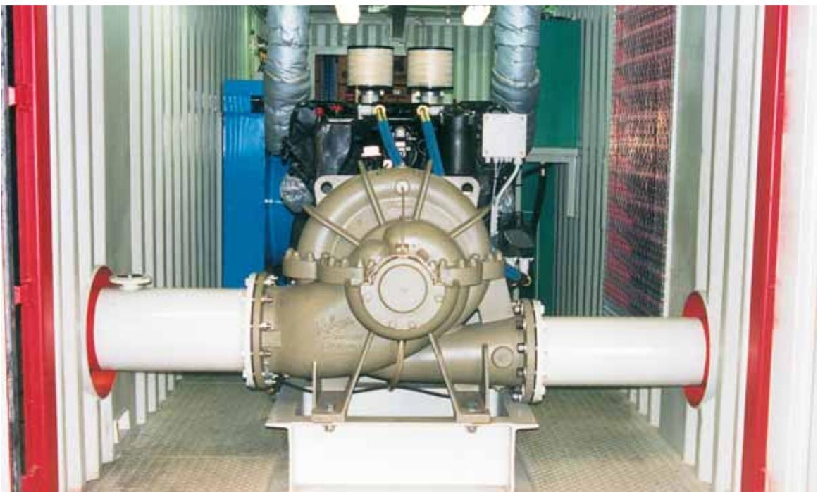
Axial split case pump with diesel engine installed in container
